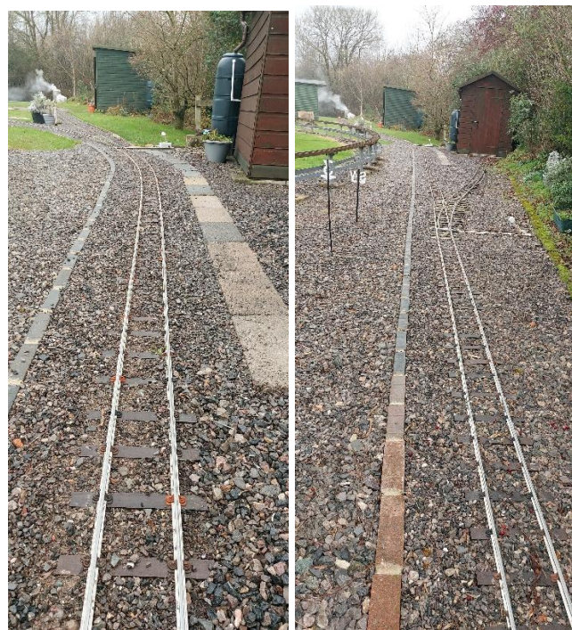
(Pic 3 & 4) Ground level ballast retaining block work, carried out by Bryon and Mike
