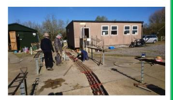
The traverser has to cross the new track and the welded steel track panel to achieve this is shown below shortly before being burried in concrete.
