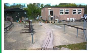
The track bed is now nearing completion and filled with ballast connecting the passing loop to the steaming bays.
