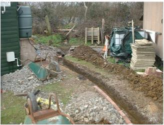
The welded track section which will soon be buried beneath the new concrete in the steaming bay apron is complete and the traverser has been modified to enable it to cross over the 5" ground level track between the steaming bays.
