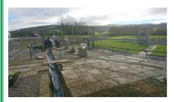
A length of land drainage pipe was laid into the trench and then connects to the existing drainage system. This will keep the new track bed drained as well as helping with the overall drainage of the site.
