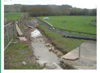
Digging the clay to lay the ballast for the track bed along the fence and around to the steaming bays highlighted the amount of water which filled the trench almost as quickly as it could be dug!
