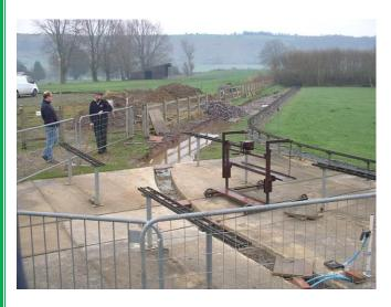
The concrete steam bay apron has been cut ready to lay the track and now joins up with the new section of track laid between the clubhouse and the workshop.
