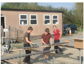
A new lifting section was also fitted to the elevated track to allow access for the lawn mower.
