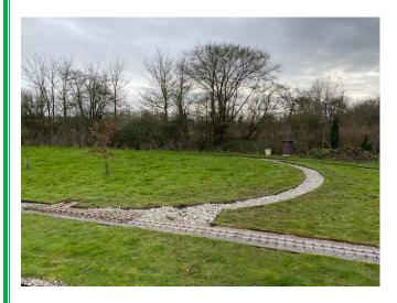
The return loop has now been dug out and filled with ballast. Ten tonnes of ballast have now been barrowed into the site.
