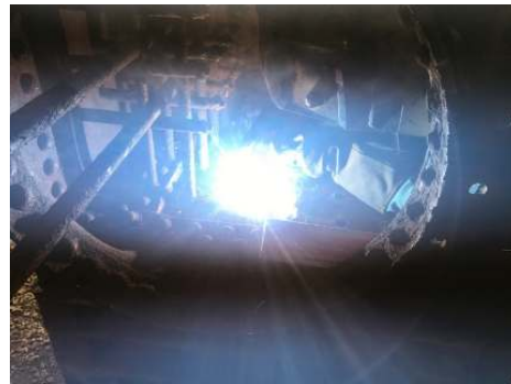
Figure 8 - Dave Goddard welding up the first set of holes
