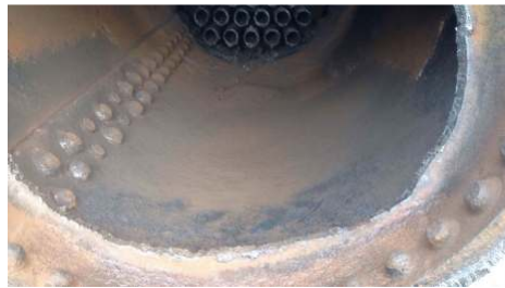
Figure 1- View of the bottom of the barrel after needle gunning
