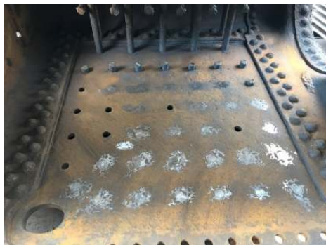
Figure 6 - Removing the stay tails to show the rings and enable centre punching
